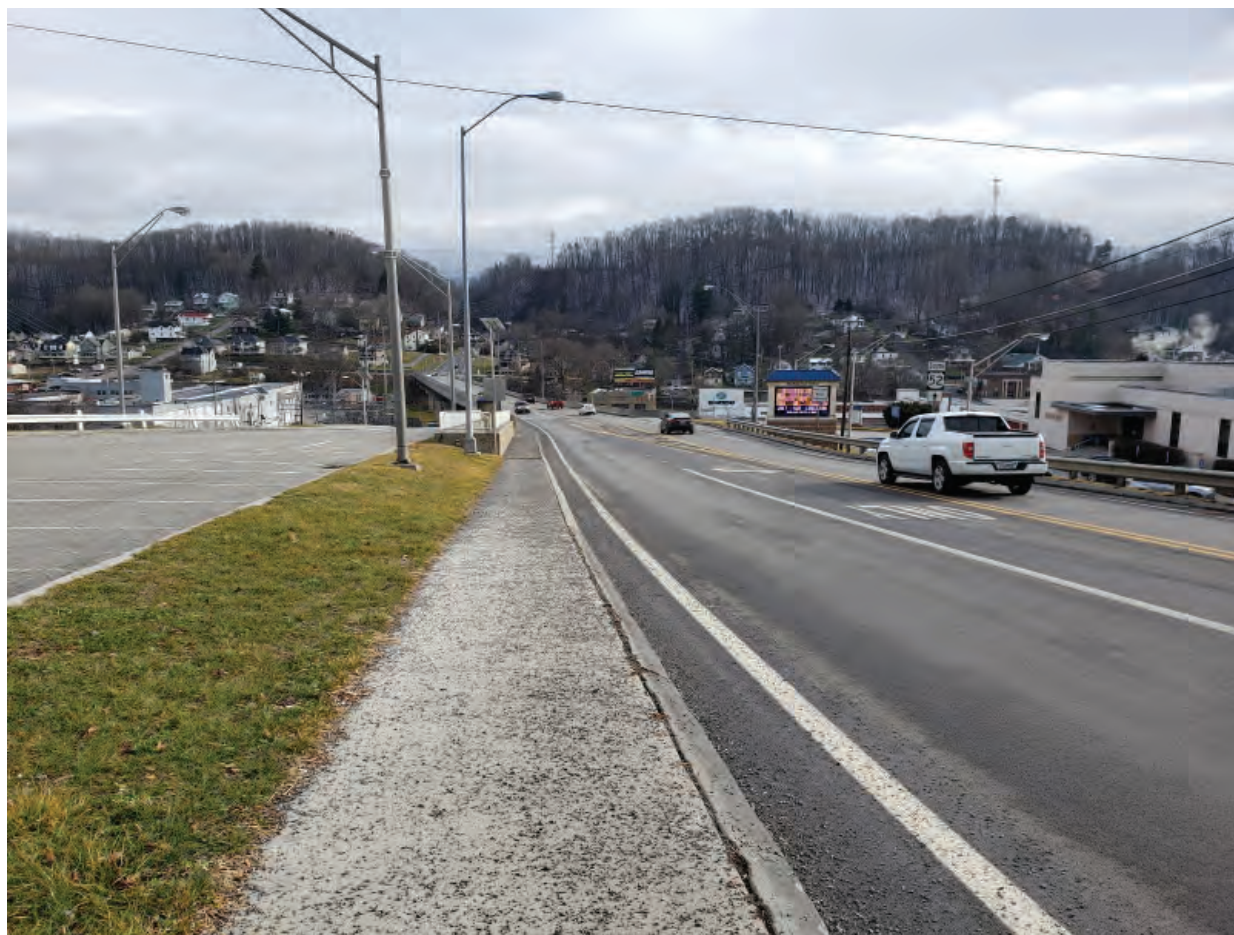
Couch Street/US Route 52 sidewalk and bridge
