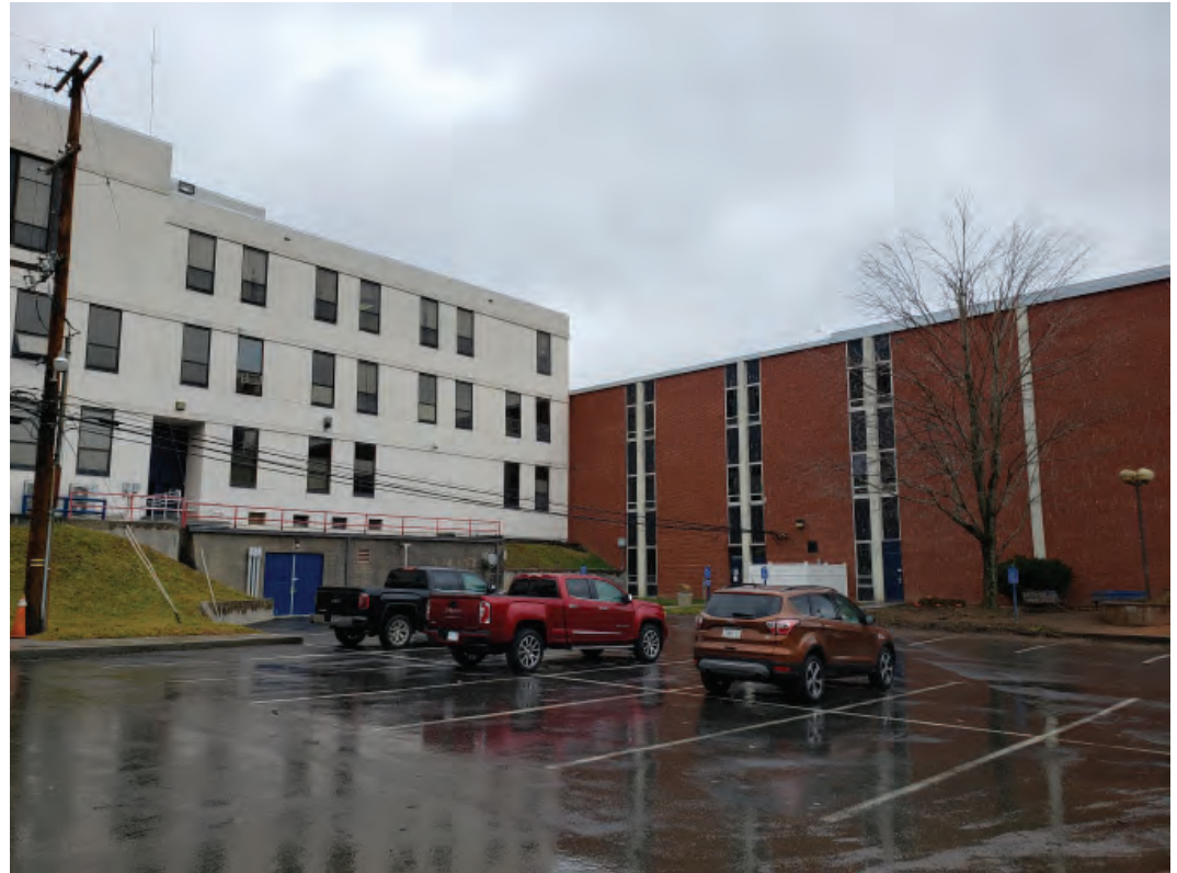
Dickason and Physical Plant (Maintenance) Building Parking
